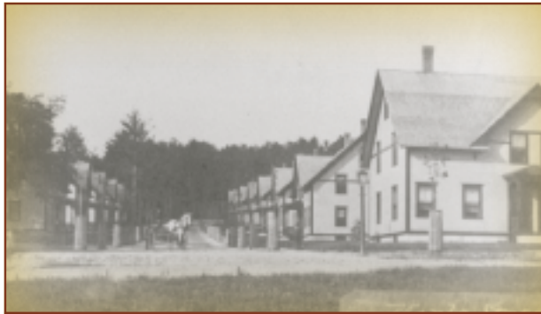
These houses for Whitin employees were built in 1889. Workers with higher status in the mill enjoyed larger, more attractive living quarters than those with lower rank. Eventually, the town contained more than a dozen clearly differentiated levels of housing.
