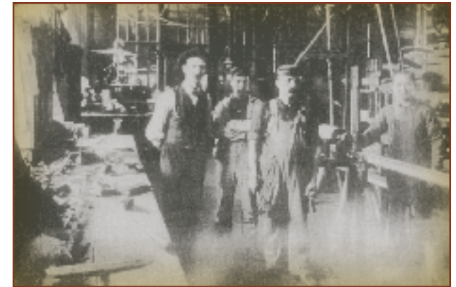
Above: Loom fixers at work. Rent for Whitin company houses in the 1860s ranged from $3 a month for an unskilled worker's multi-family house to $12 a month for a single family upper-level manager's house. The average weekly pay was around $6.60 for a 60-hour week.
