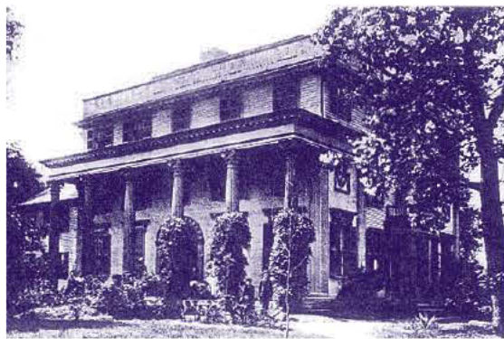
Asa Waters II spent two years gathering materials for his "honeymoon cottage," shown here in the 1880s. It was one of the last buildings in town to use the Georgian Colonial design. Materials in the house include Southern hard pine and brick, Central American mahogany and Italian marble. The woodwork was handcrafted and the house designer, Asher Benjamin, was brought in from Boston.
