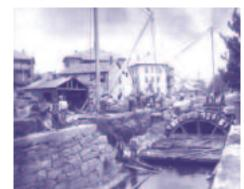
When the Blackstone Canal Company folded, parts of the abandoned trench deteriorated into rank open sewers. During the 1890s, they were sensibly integrated into Worcester's underground waste water system. Dressed granite blocks from the 13-foot walls of the 82-foot long locks were sold and carted away to become parts of new buildings. During deep excavations, the city's highway department even now sometimes uncovers the canal.
